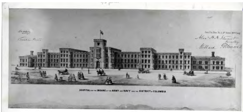
Fig. 6: Saint Elizabeth's Hospital Predecessor Institution—The Government Hospital for the Insane
